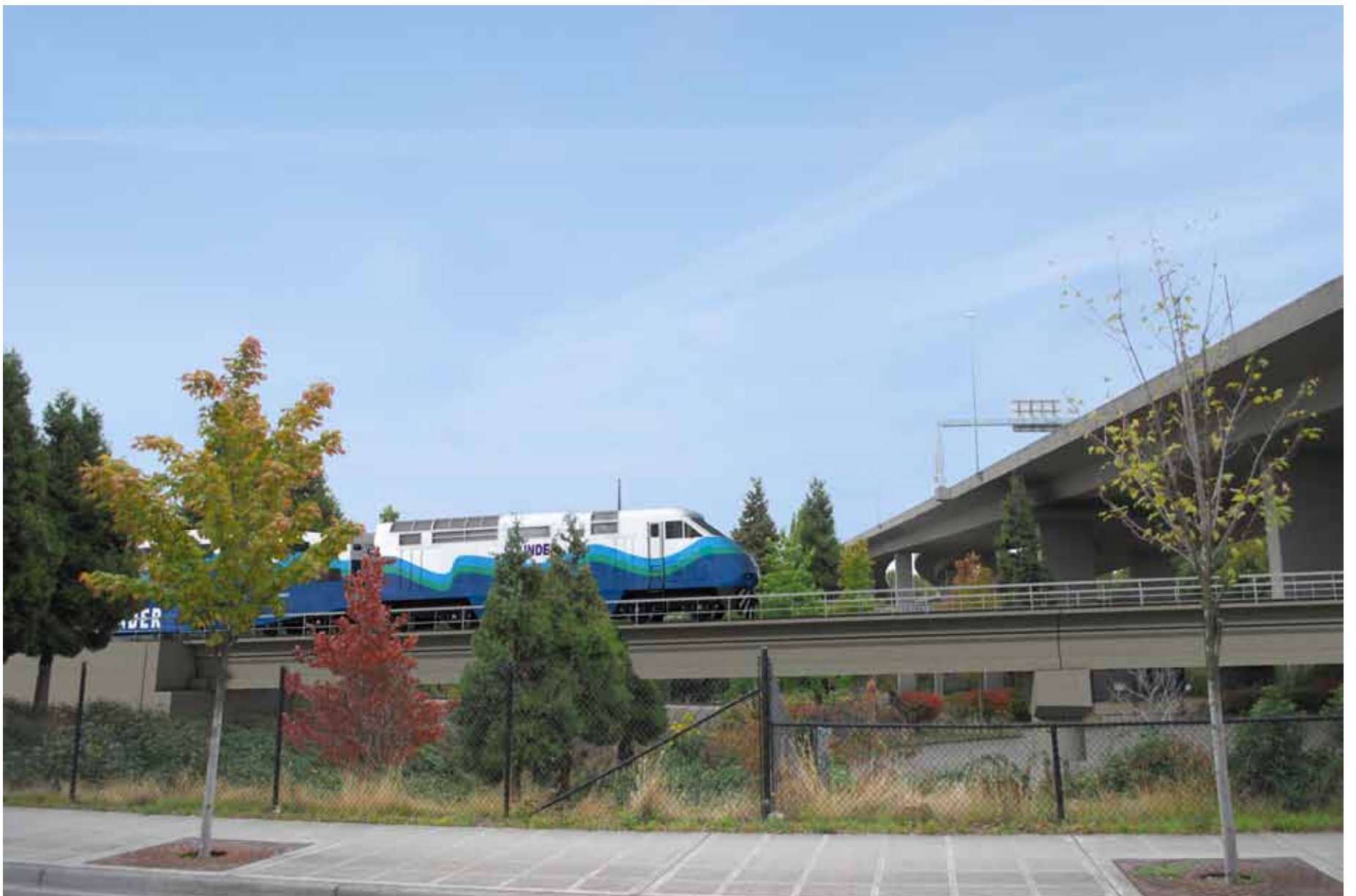
'B' Street Gully Bridge, looking south from East 25th Street
