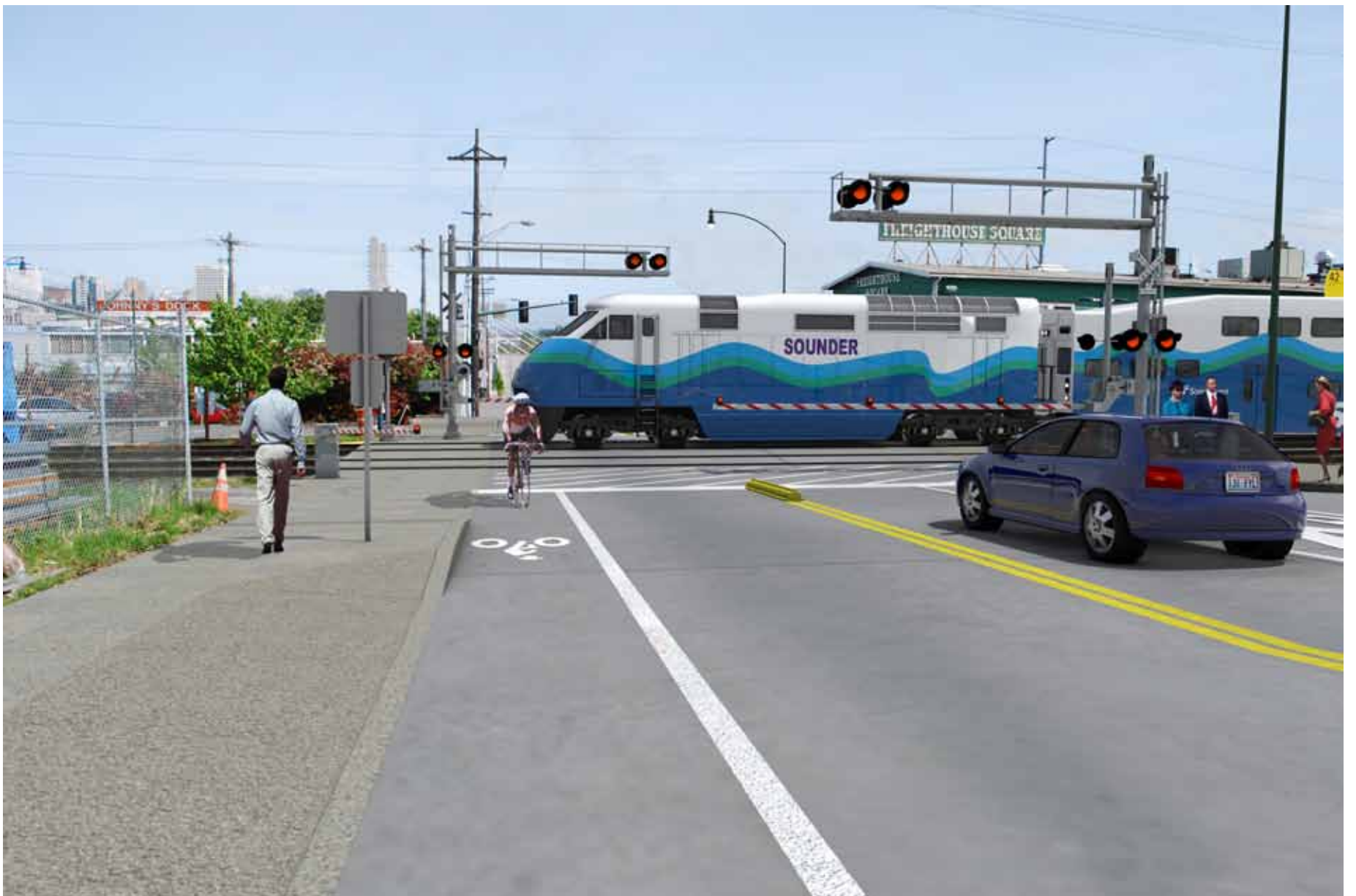
East D Street crossing, looking north from East 26th Street
