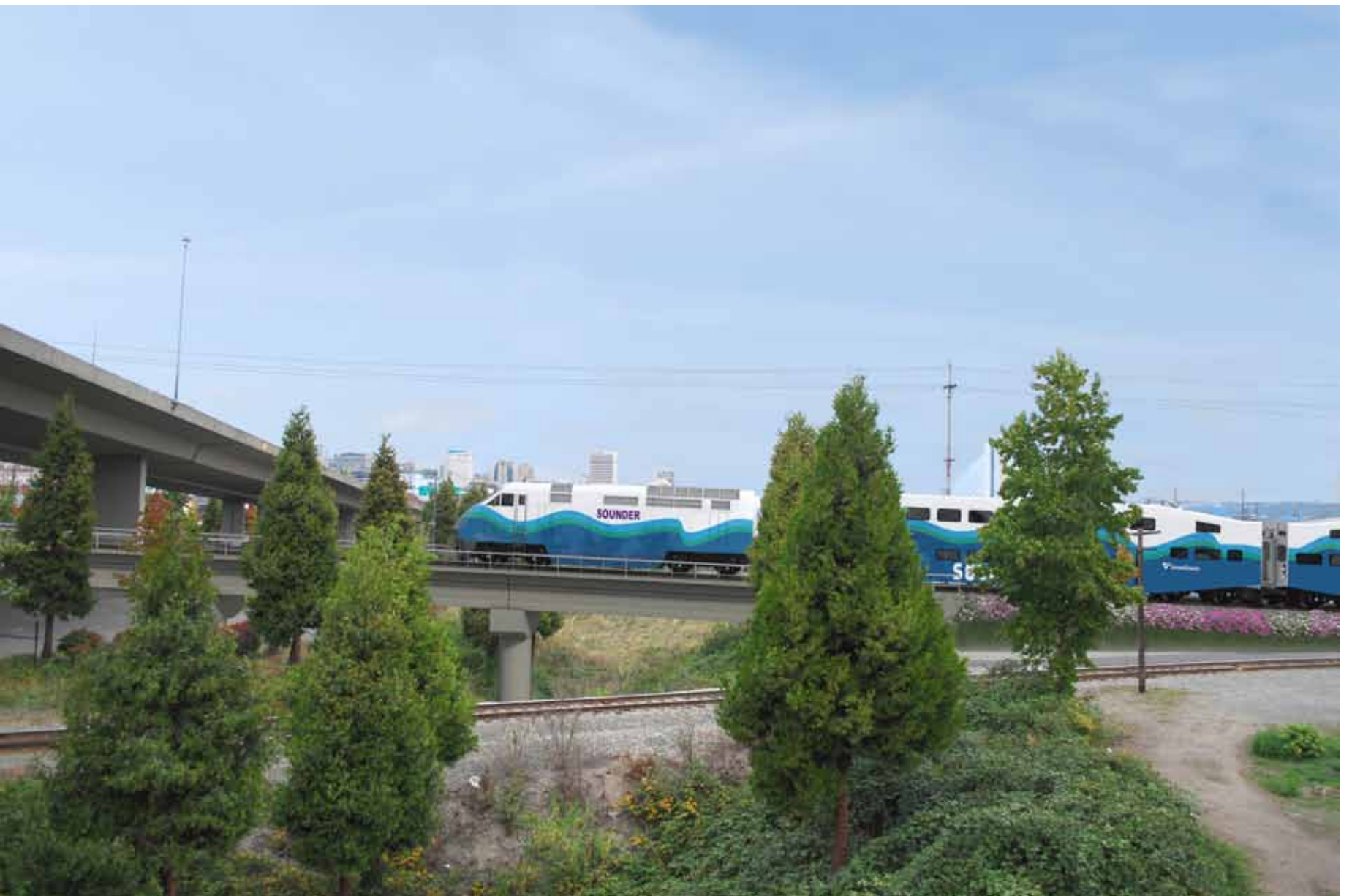
'B' Street Gully Bridge, looking north from East 26th Street
